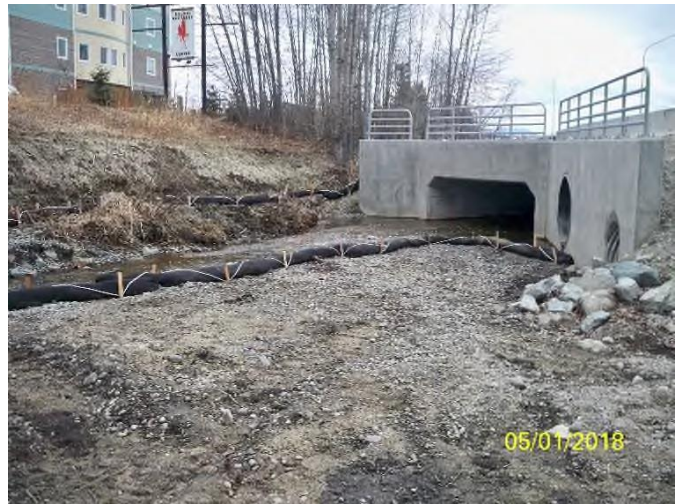
North Fork Little Campbell Creek box culvert with down-slope sediment control measures. (DEC Photo 24)
